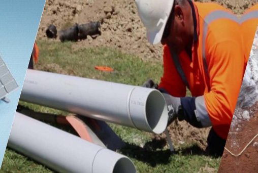
Underground Water Supply Pipe Line
