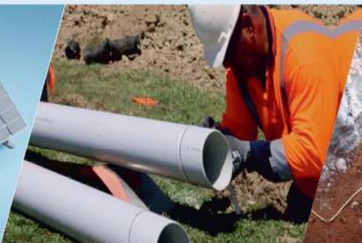
Underground Water Supply Pipe Line
