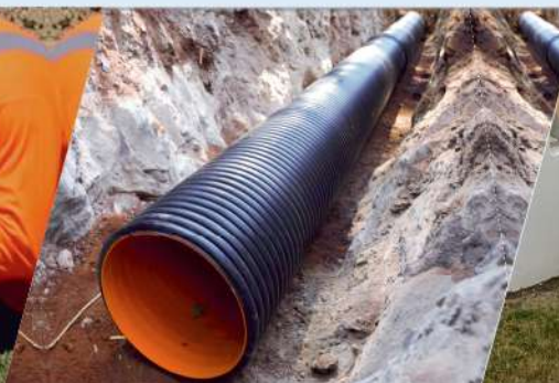
Underground Sewer Pipe Line
