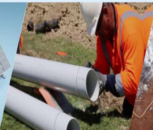
Underground Water Supply Pipe Line
