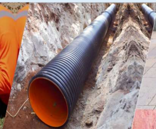
Underground Sewer Pipe Line
